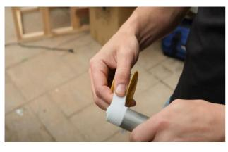
Wrap 3 layers of thread tape around the threads on both ends of one of the long pipes.
