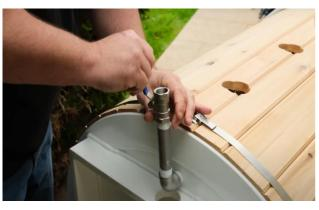
Screw the valve onto the end of the long pipe.
